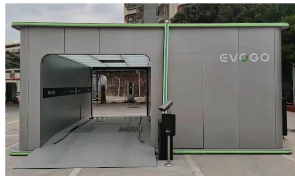
Figure 9: EVOGO battery swapping station, Source: EVsmartBlog
